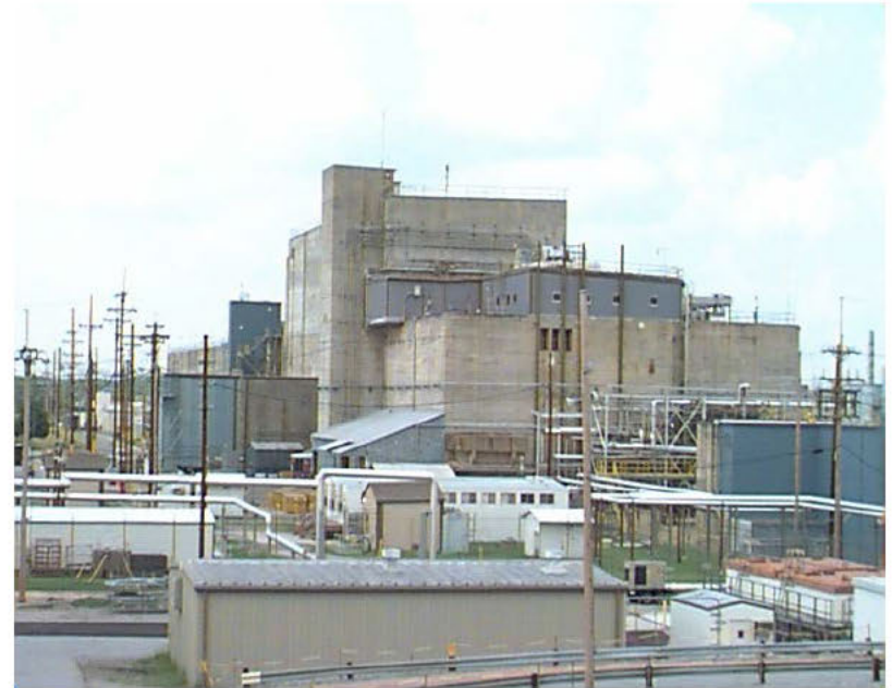
View of H-Canyon/HB-Line (looking North)
